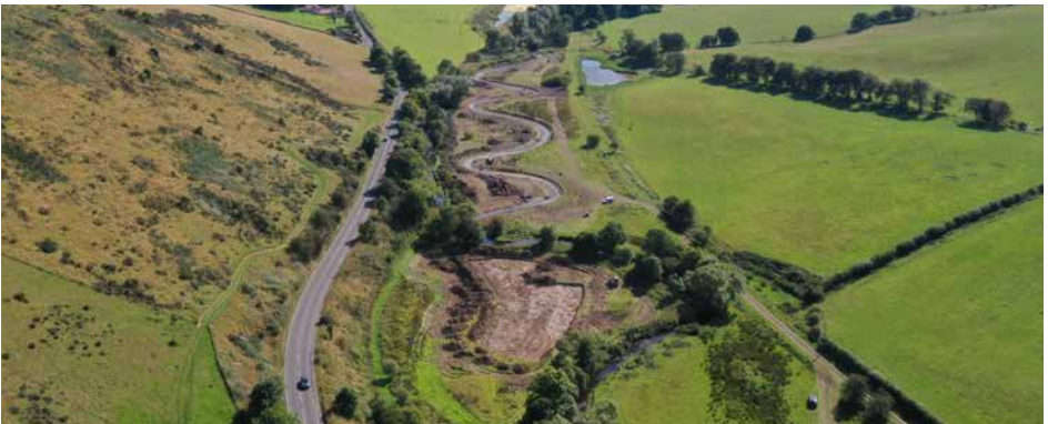
The restoration works at Nether Kidston get underway
