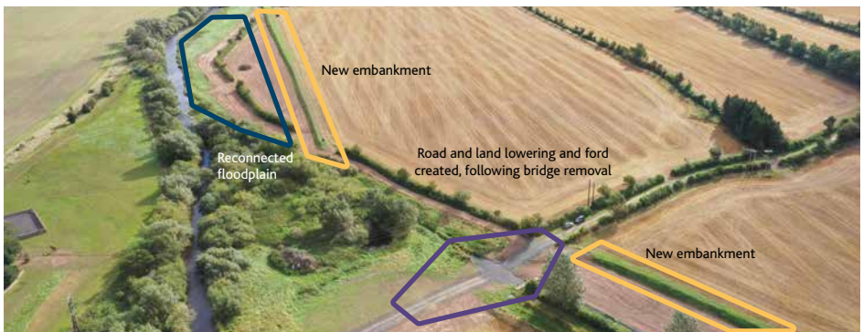
Detailed look at the restoration works around Coupland Bridge on the River Glen
