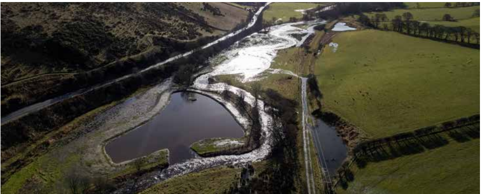
The completed restoration works at Nether Kidston after a small flood
